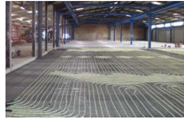
New heating in Hall 2 (Hot water underfloor heating)
