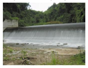
power plant where Kubota's small-sized hydraulic power generation system was adopted, 70kW of electricity are generated using water of the Mon river, a branch of the Mekong river. In this way, electric power is supplied for 24 hours a day to about 350 households in seven villages. So the plant is useful to improve the standard of living of people without environmental load.
