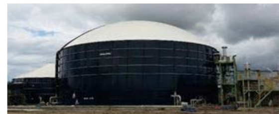
First palm oil mill effluent processing facility in Malaysia (for BBC Biogas) External view of membrane-type methane fermentation facility
